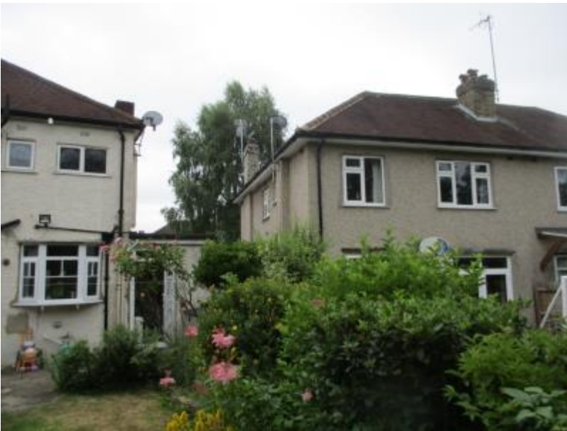
Looking towards rear of 51
