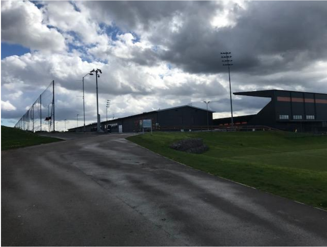
Existing north and east stands
