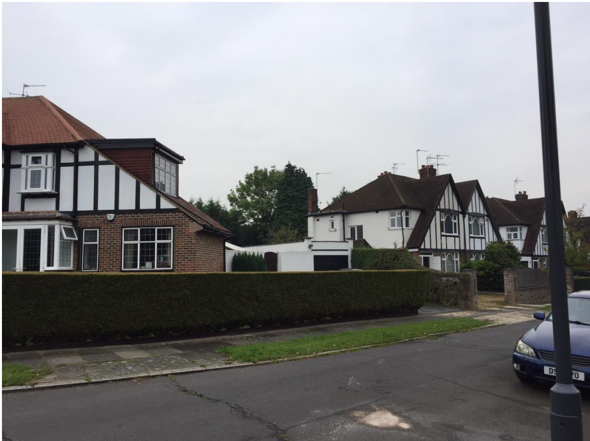
Front/side elevation of host dwelling when viewed from Furham Feild
