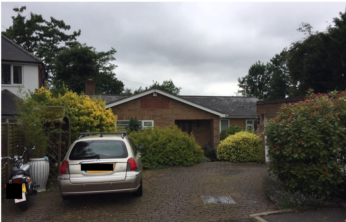
Existing front elevation of the subject property and detached garage, and the neighbouring property No.5a Crest View located to the left.
