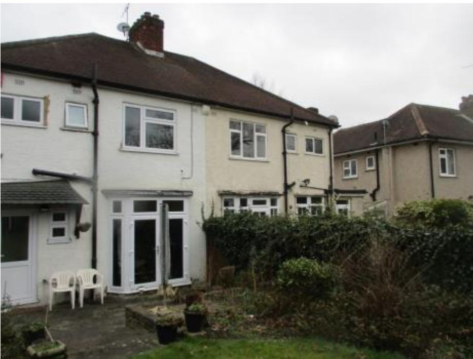
Looking towards rear of 53
