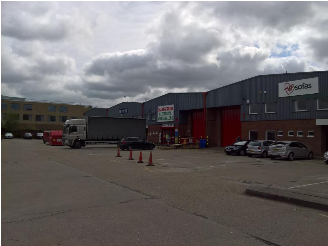
Application unit at top centre
